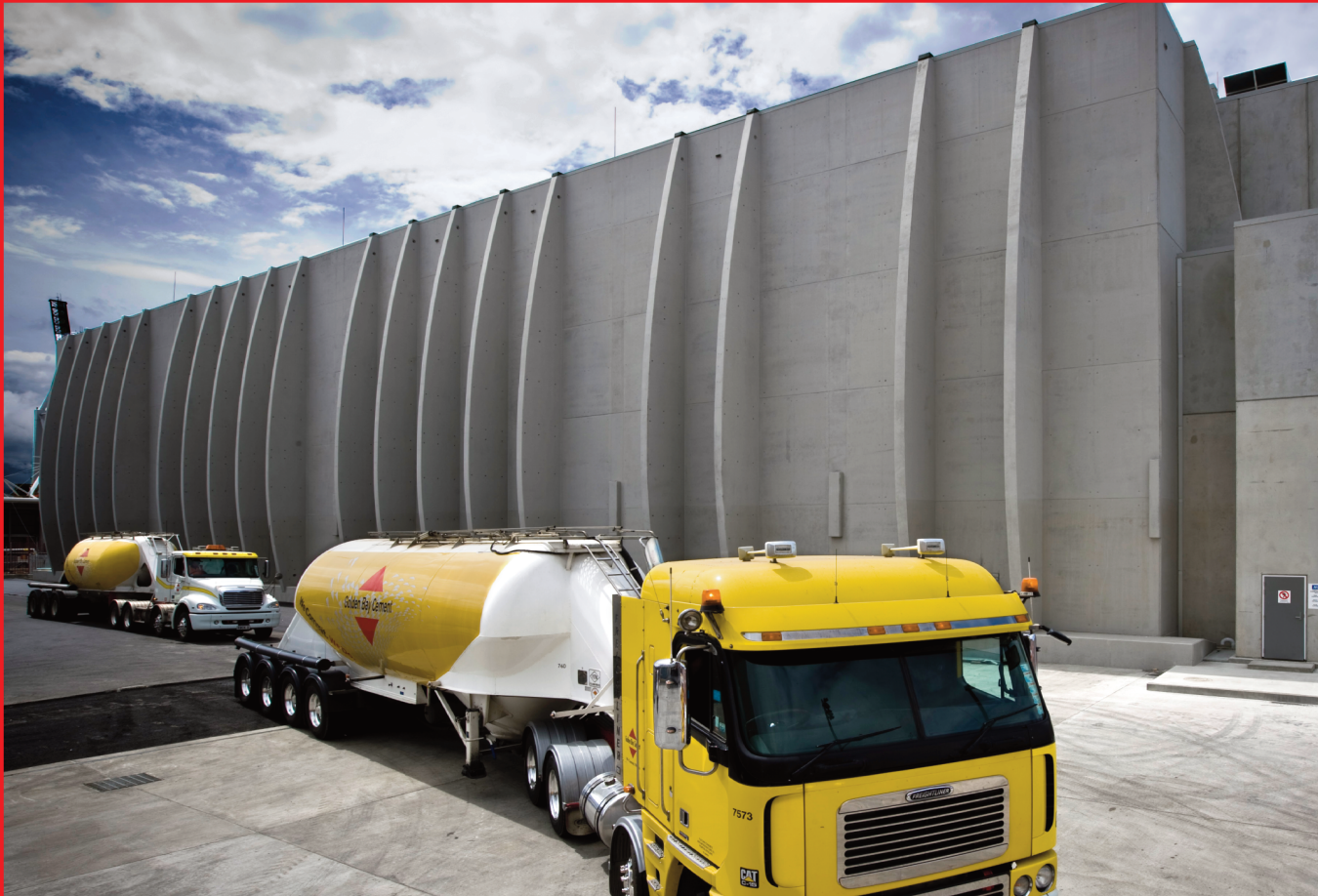
Flat Storage Hall Terminal for Golden Bay Cement / Fletcher Construction, Auckland, New Zealand
