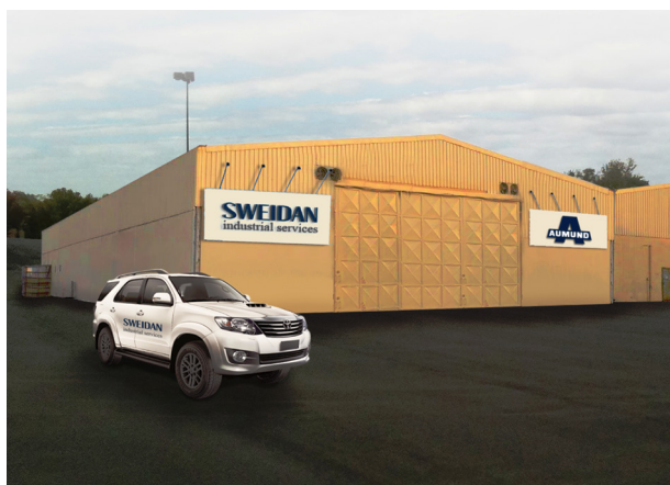
The new SWEIDAN and AUMUND warehouse at Riyadh
