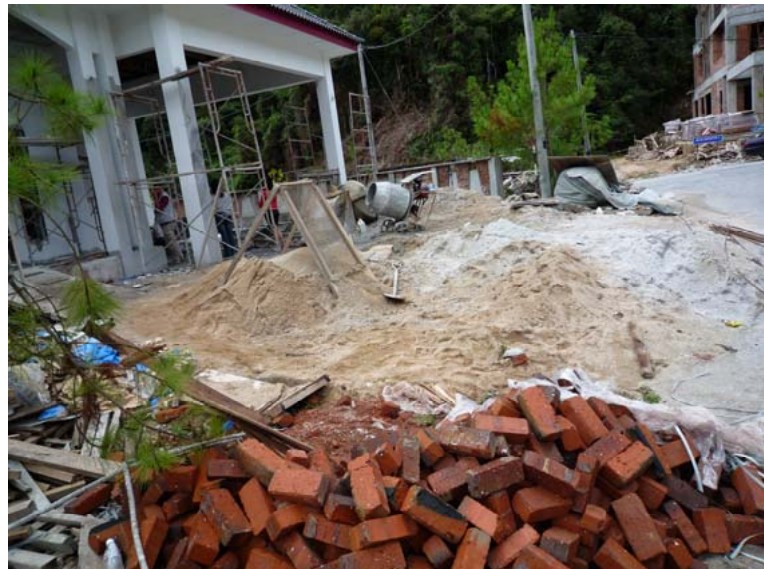
Figure 1: Conventional jobsite in Borneo (Malaysian part)
