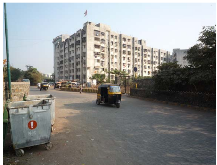
Figure 2: Cracking and water damage on a residential complex in Mumbai
