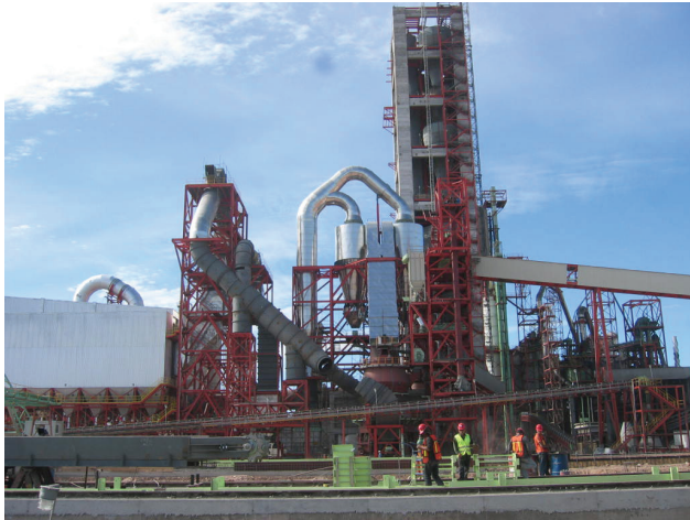
A LOESCHE mill of type LM 46.4 in the Yaqui cement works in Mexico.
