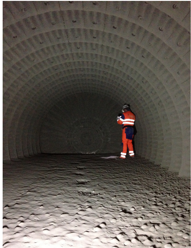
Figure 3 – GCP Applied Technologies employee during a mill audit
