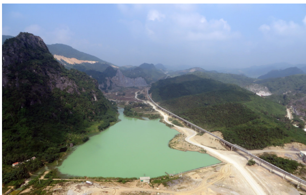
Figure 3: BEUMER managed to route the conveyor along a very narrow stretch of land in Vietnam for the cement producer Cong Thanh
