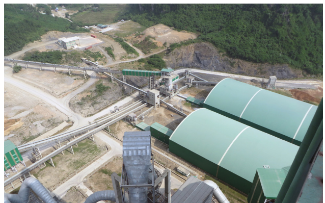
Figure 4: Transfer situation before the blending bed
