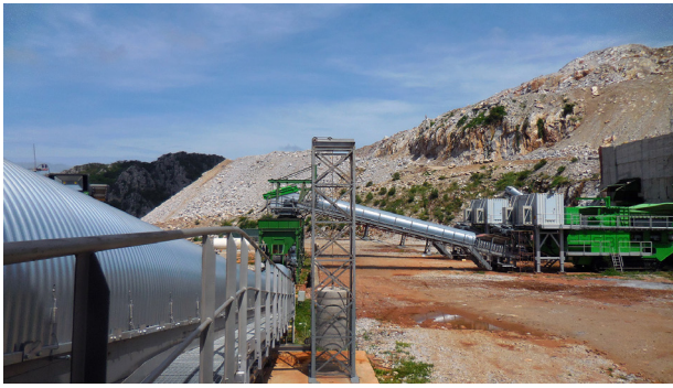
Figure 2: Transfer tower in the feed area
