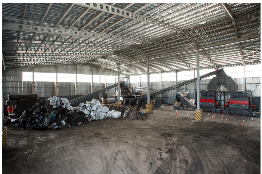
RDF Plant Adana, Turkey
