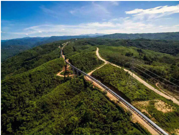
Figure 5: The route of the overland conveyor for the end customer, Cemindo Gemilang, passes through the middle of the rain forest
