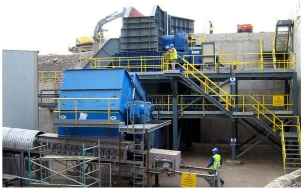
Shale Sizer Installation – Irish Cement
