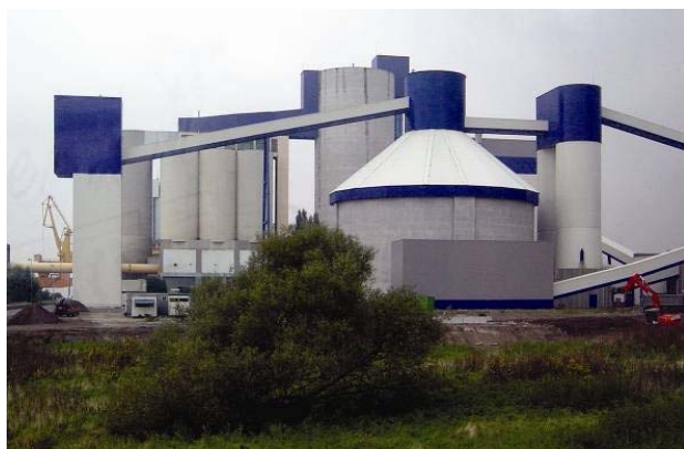
CBR Ghent Silo Storage System
