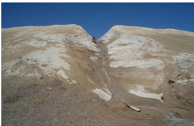
Fig. 7: CKD dumps slope stability issue
