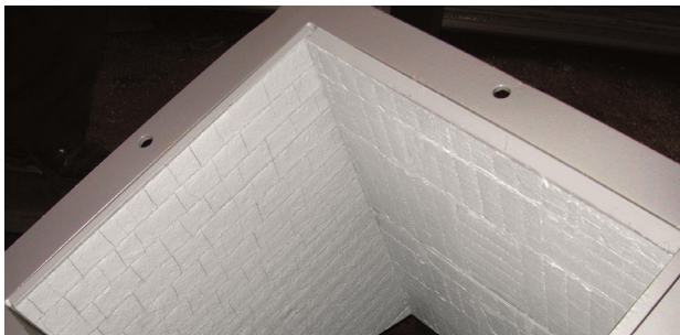
Figure 5 KERAFLEX lining of a bunker that is exposed to high sliding and impact wear. Moreover, the system allows significant noise reduction.
