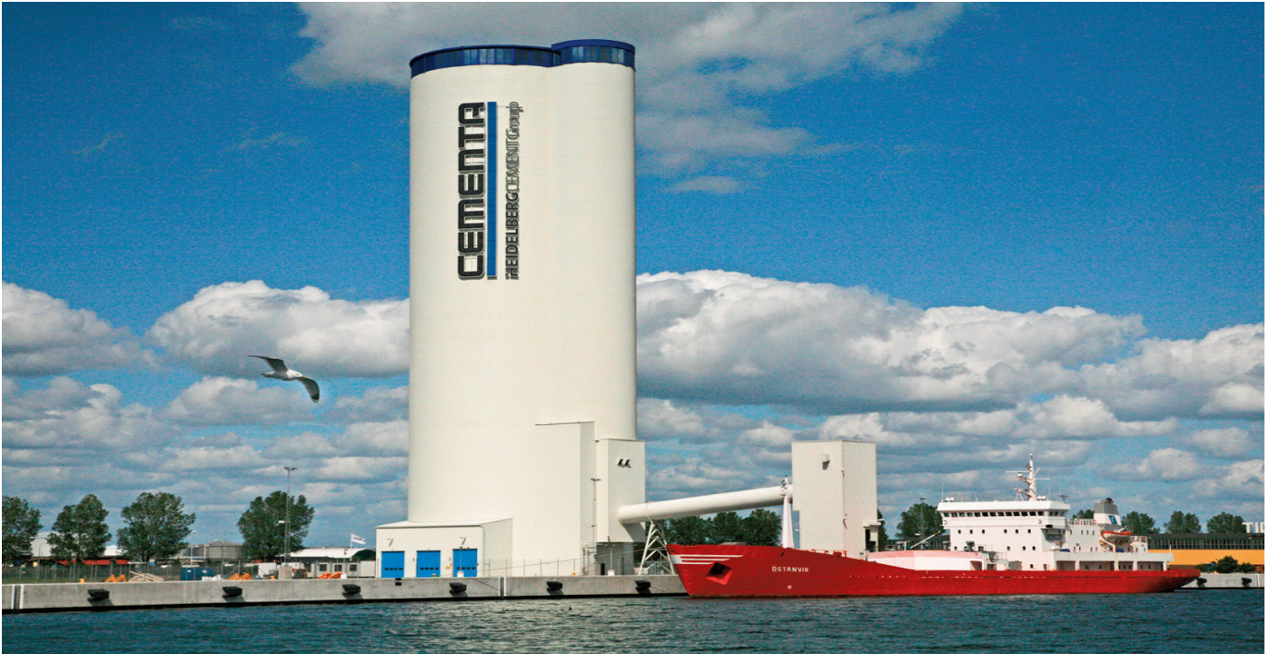
EXAMPLE MALMÖ/SWEDEN: The worlds largest multicompartment silo, with a capacity of 30.000 t, diameter of 26 m, height of 90 m, built for CEMENTA AB HeidelbergCement Group, commissioned in 2011 after only 18 months, without any delay or accident.
