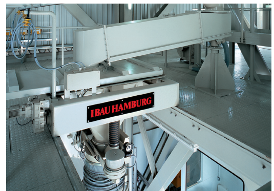
Bulk loading with IBAU Simplex loader
