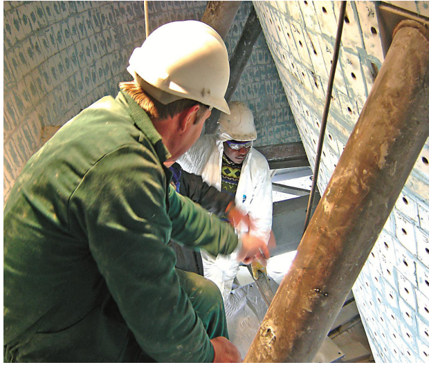
Figure 6 KALOCER high alumina ceramic lining in the separator zone of a vertical roller mill.
