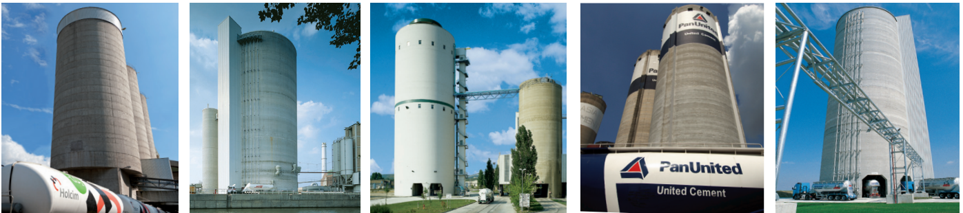
MULTICOMPARTMENT SILOS FROM IBAU HAMBURG: The base of the silo floor is formed by the central cone which has proven its worth over many years in ring silos. The compartment divisions result in clear external diameters of 14 to 27 m.
