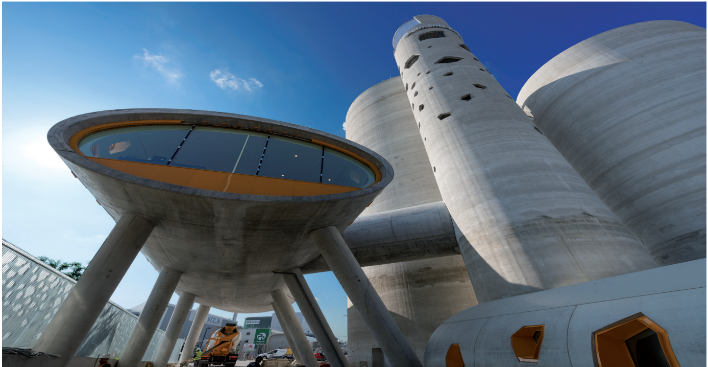
IBAU's newest Multicompartment silo in Paris/France built for Ciments Calcia / Semapa and inaugurated on 4 th July 2014.
