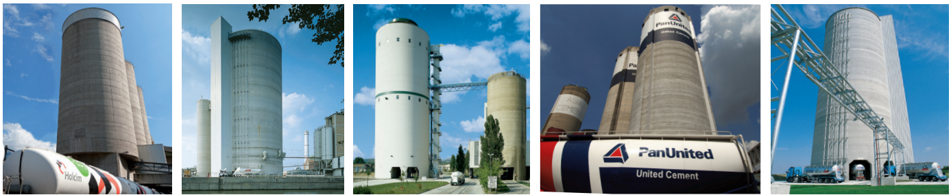
Multicompartment silos from IBAU HAMBURG: The base of the silo floor is formed by the central cone which has proven its worth over many years in ring silos. The compartment divisions result in clear external diameters of 14 to 27 m.
