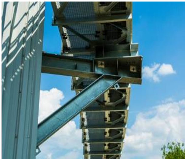
Picture 4: The first support is mounted directly to the storehouse.
