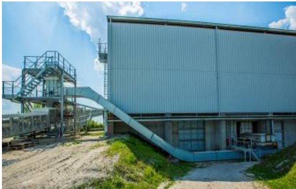
Picture 3: The chain belt conveyor lifts the material to the height of the Pipe Conveyor.
