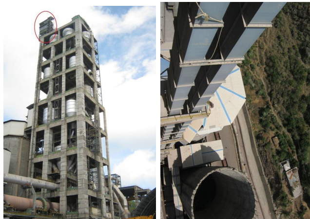
Fig 4) Belt bucket elevator for feeding the heat exchanger of a rotary kiln feeding cement silos (Lafarge Wössingen)
