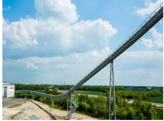
Picture 5: The inclination of the Pipe Conveyor measures 18.6 degrees at the point shown.
