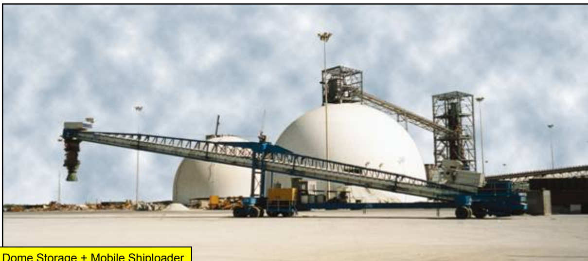
Dome Storage + Mobile Shiploader
