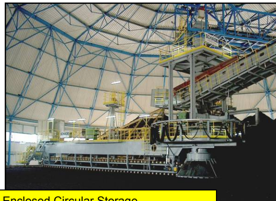
Enclosed Circular Storage
