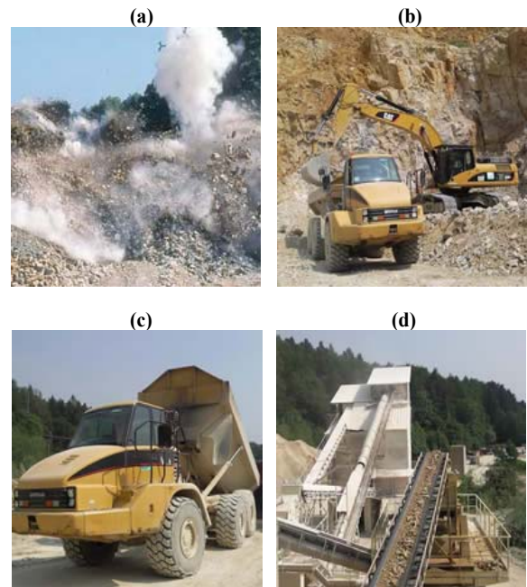
Figure2: exploitation of a career. (a): slaughter of the rock by blasting; (b): loading of excavated material; (c): transport of the material by dumper; (d): crushing of the material
