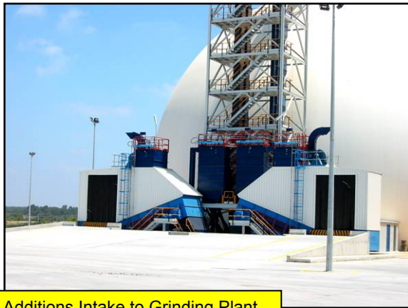
Additions Intake to Grinding Plant
