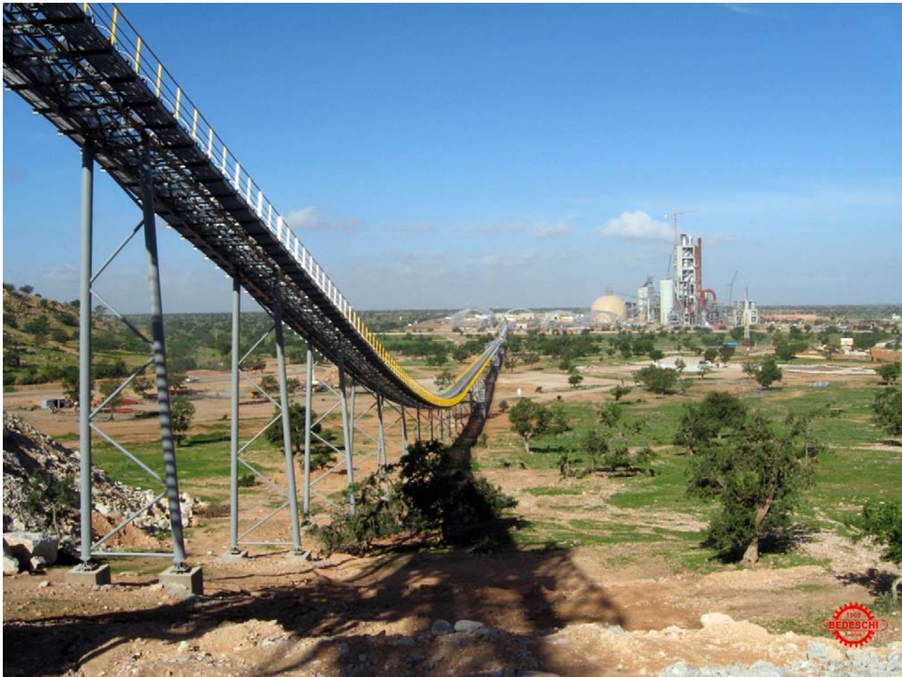
Fig.5 Ait Baha Cement Plant
