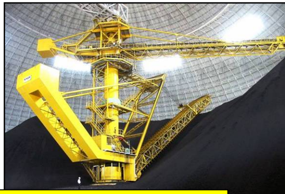
Circular Storage 120 metres diameter
