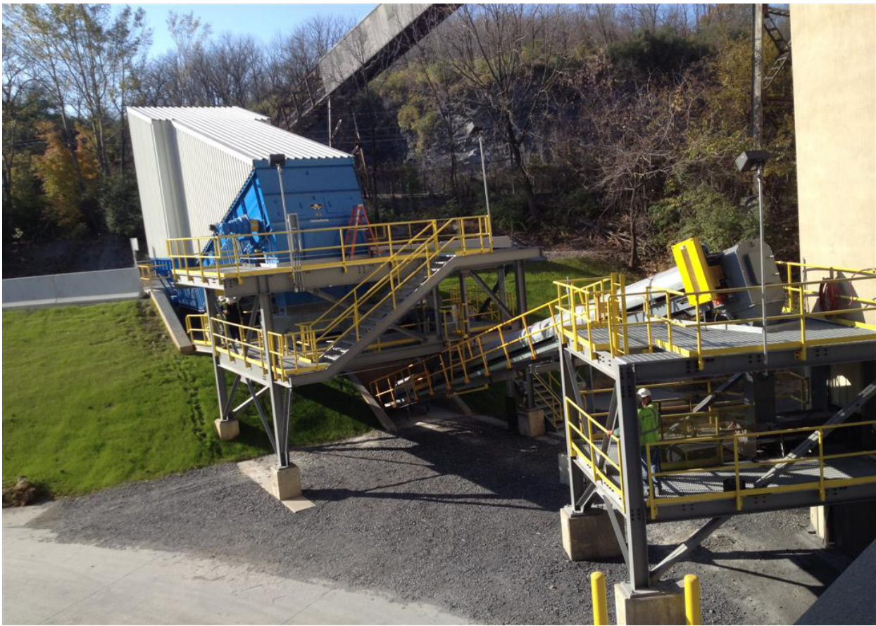
Cap 2) Multiple Samson® Storage Feeders at Lehigh Cement (©2014 AUMUND)
