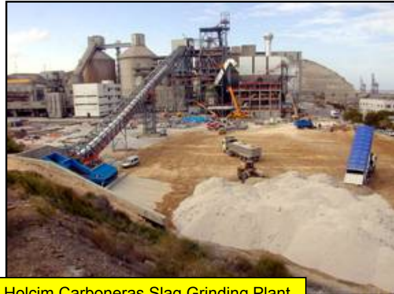
Holcim Carboneras Slag Grinding Plant
