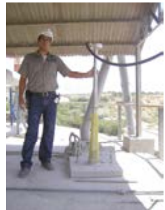
Cleaners PAS 75 S acoustic cleaner installed on a 8000 tonne cement silo in Haiti
