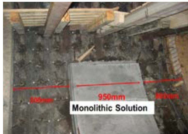
Picture 2: Tire section in the upper transition with a monolithic lining
