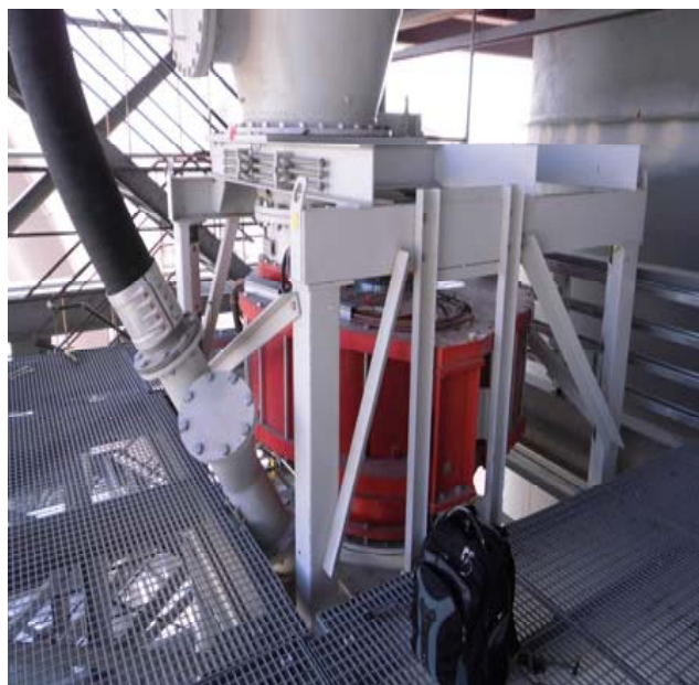
Pic 3: The red rotor weighfeeder Pfister® TRW-S/D is designed to dose up to 12 t/h of alternative fuels at Arabian Cement
