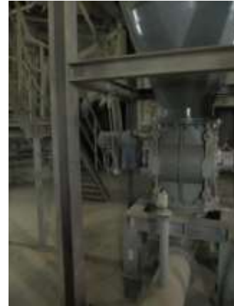
Figure 18: Fly ash rotary valve
