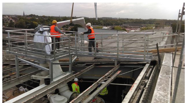
Figure 2: Installation of an explosion vent by Thorwesten Vent personal.
