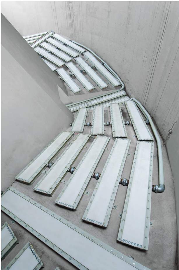
Figure 2: Silo bottom of central cone silo
