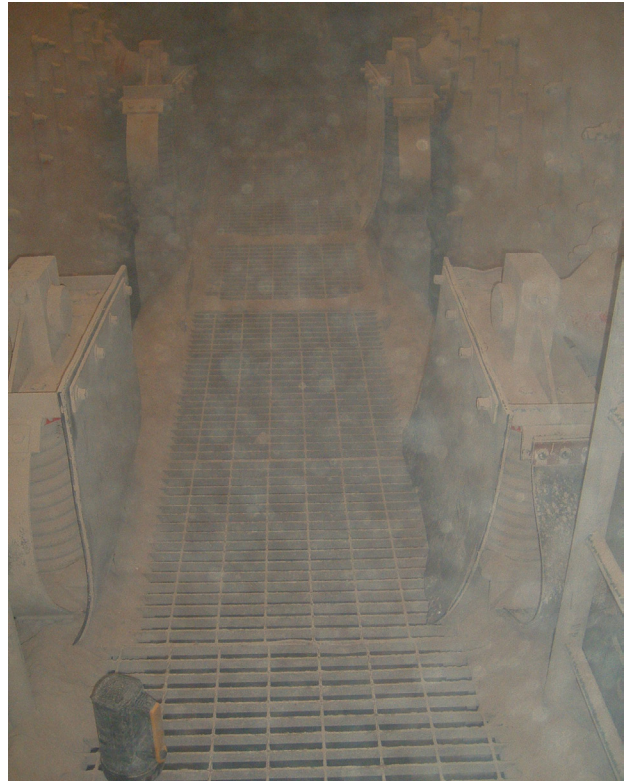
Hycontrol Screenhouse Interior
