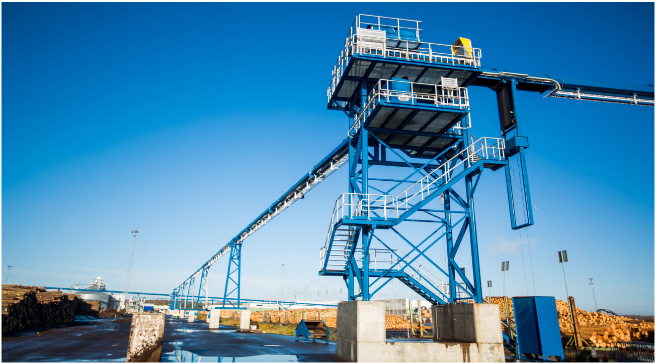
Picture 2: The fully enclosed system is particularly suited to the safe transportation of dust-laden materials.
