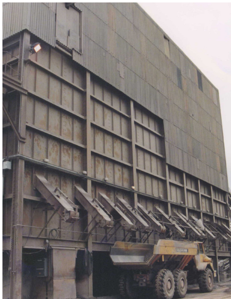
Hycontrol quarry screenhouse
