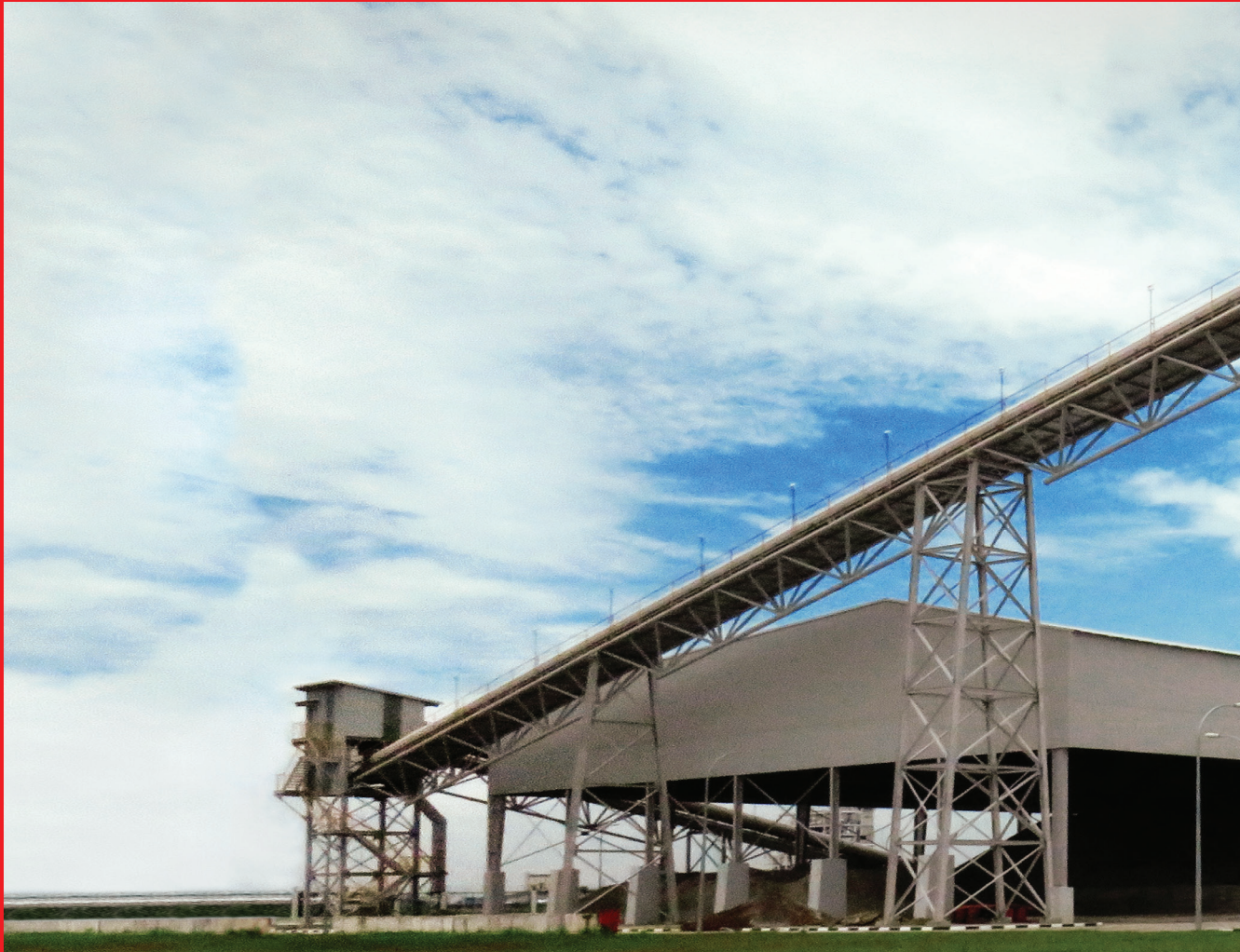
Blast furnace slag silo plant of Meridian Maplestar Sdn. Bhd., Malaysia with IBAU Gdischarge System
