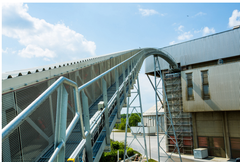
Picture 1: The alternative fuels are conveyed from the storage to the main burner, low in noise and dust-proof.
