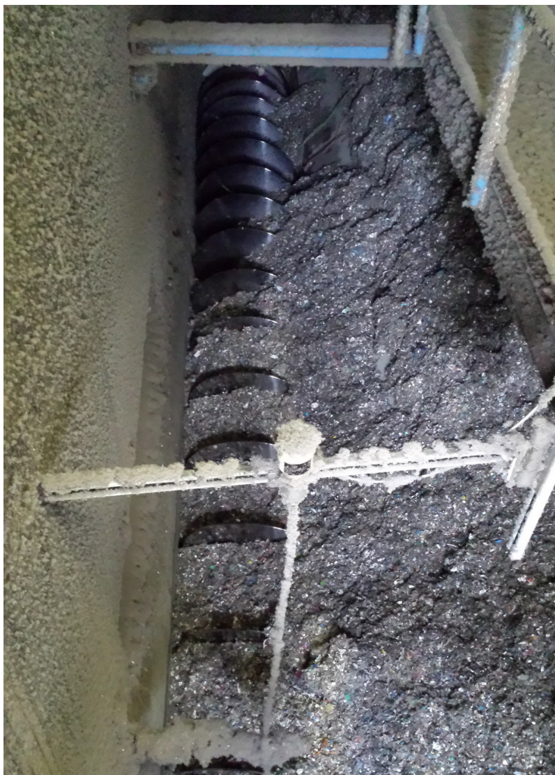
Picture 3: Fill level measuring probes and other measuring technology monitor the automated processes.
