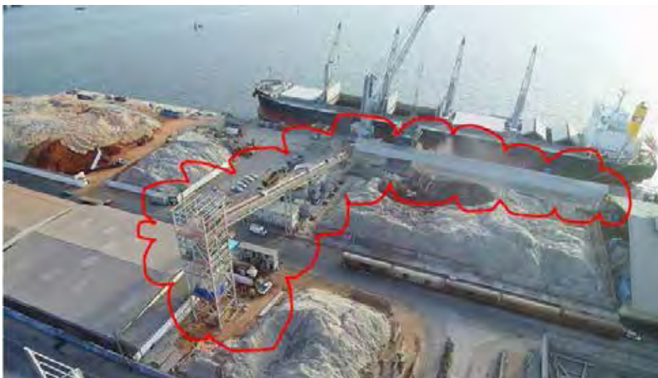
Ship unloading system for Sea Invest in Abidjan successfully commissioned and handed over in Q4/2017
