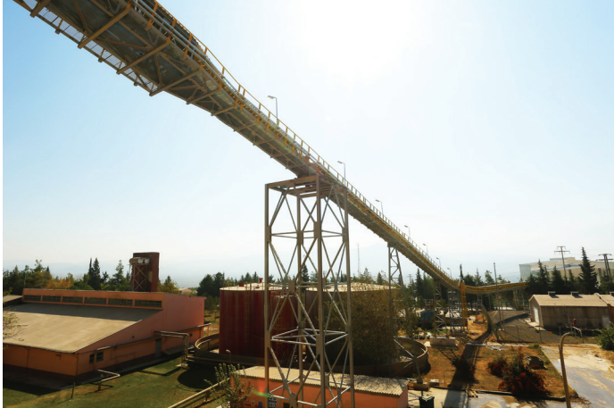
Picture 4: With its ability to navigate horizontal and vertical curves, the conveyor can be optimally adapted to the terrain.
