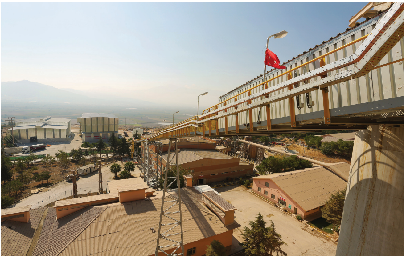
Picture 3: The Pipe Conveyor transports the alternative fuels from the storehouse to the preheater.
