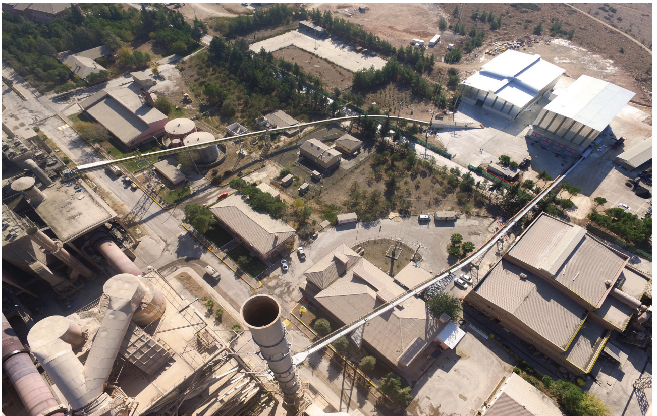
Picture 6: Two successive conveyors, 206 and 190 metres long, are used. Each Pipe Conveyor reaches a capacity of 15 tonnes per hour.
