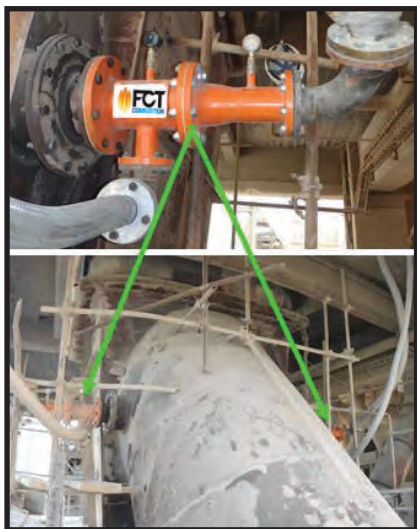
Figure 5: Installation of the FCT burners in the TAD.
