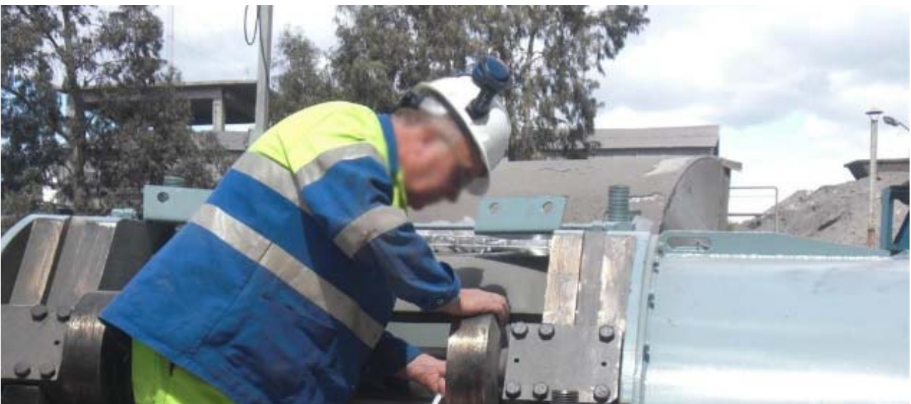
Fig 9 –Kiln upgrade with Bogiflex® KGD26
