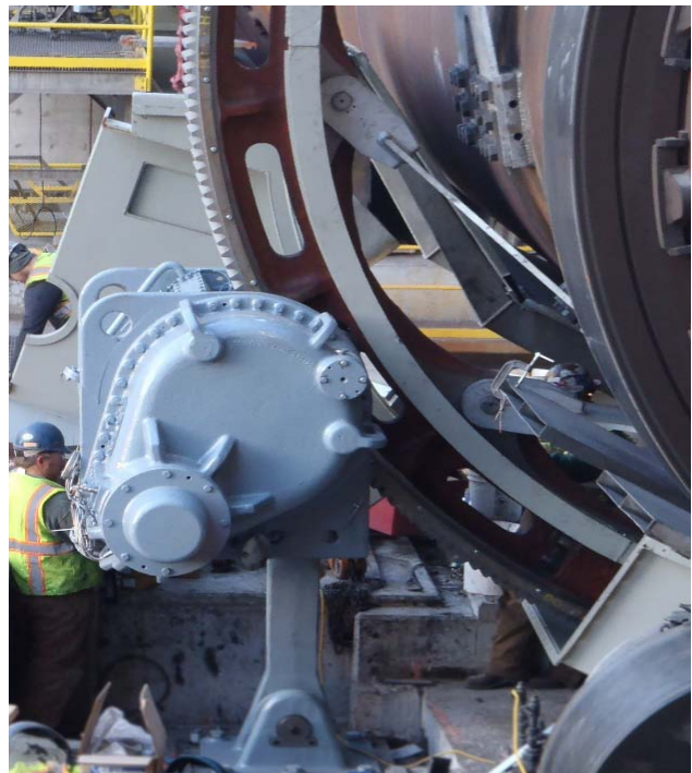
Fig 10 – example of Bogiflex® KGD20 during installation
