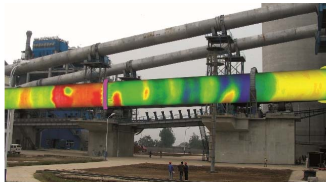
Fig 2 – Thermal readings of running kiln
