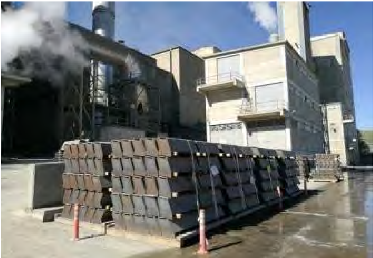
Photo 2: The narrow and weight-reduced design of the GSZF reduces the costs for steel structure and freight. The operator was able to save considerably on costs.
