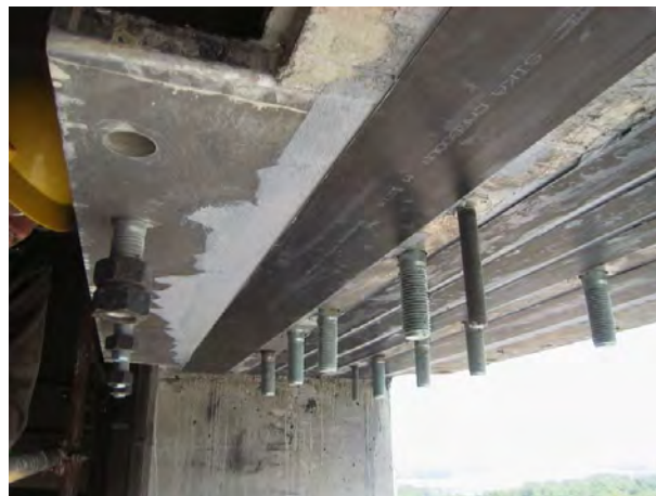
Figure 8: Beam and anchorage plate during strengthening
