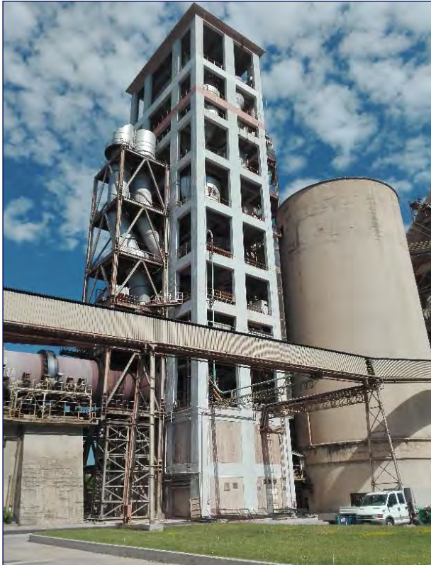
Figure 2: View of the cyclone tower
