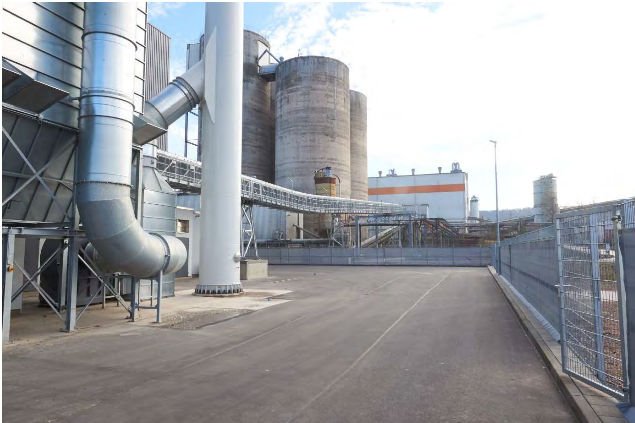
The 420-metre-long pipe conveyor at B+T Deuna connects the SRF facility with the cement works, making it crucial to the plant's success.
