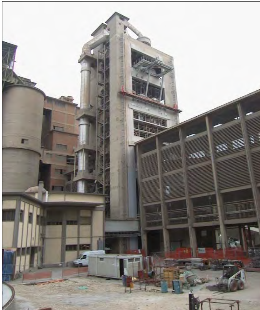
Figure 6: View of repaired cyclone tower
