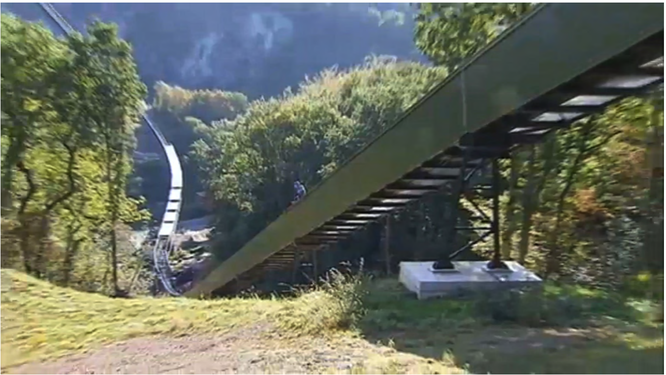
Picture 6: Direct routes can be realised, among other things up and down steep hills. The systems can overcome large inclines and gradients.
