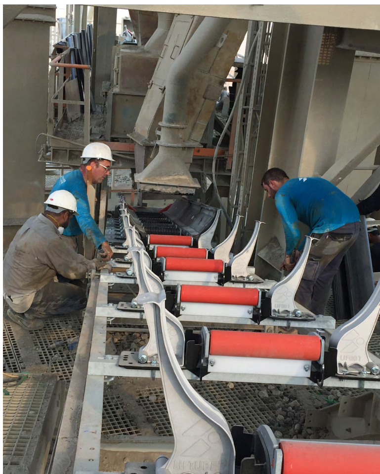
1-Liftube installed on Crusher falls conveyor
