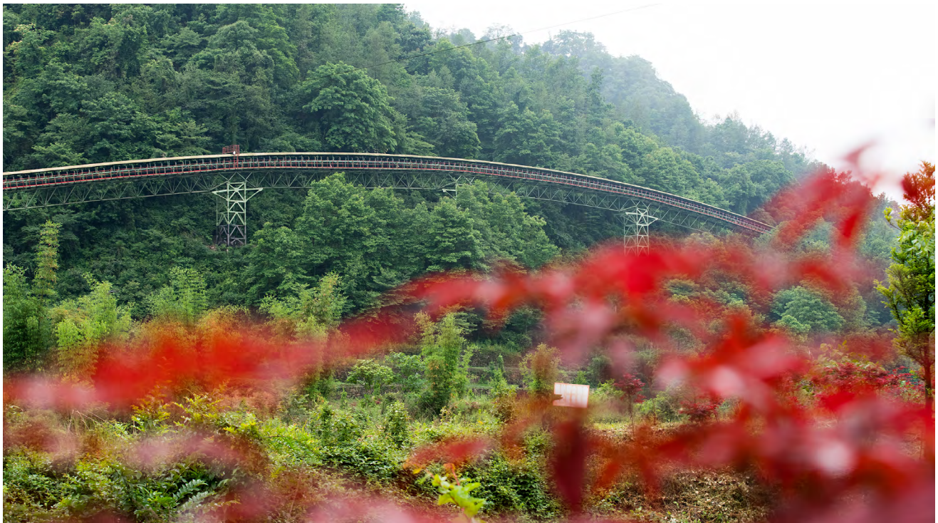
Picture 2: Sichuan project: whenever technically possible, the routing of the conveyor has been adapted to the topography.
