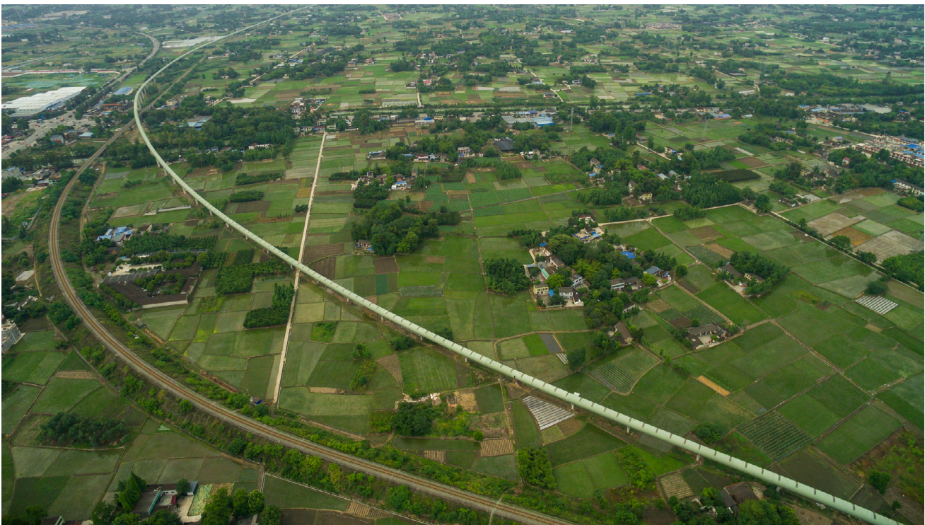
Picture 1: Project Sichuan: BEUMER Group built a 27 kilometre long conveyor system through hilly terrain and unstable ground.
