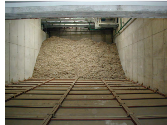
AUMUND Moving Floor type SBA
