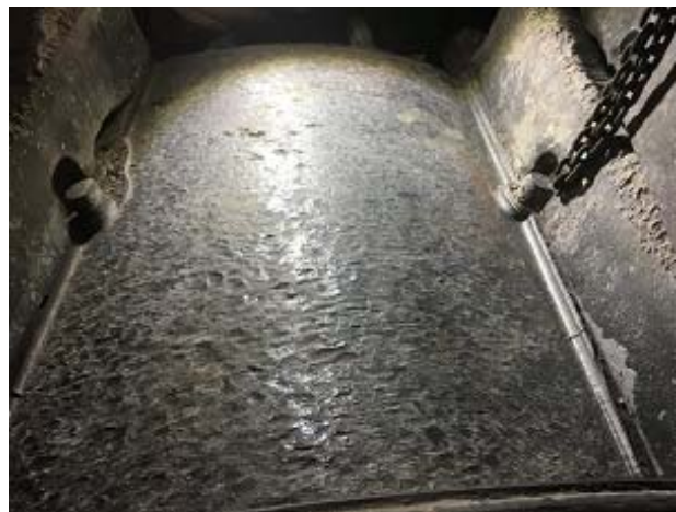
An aggressive wear is appear on the roller hub surface.
