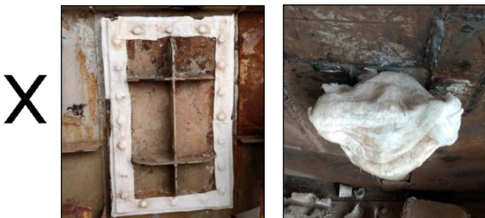
Fig 05: Conventional False Air arresting methods (By Ceramic Paper + Sodium Silicate)
