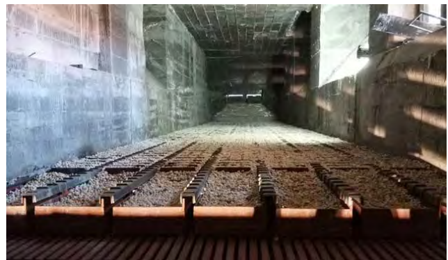
View into an ETA cooler including the autogenous layer.
