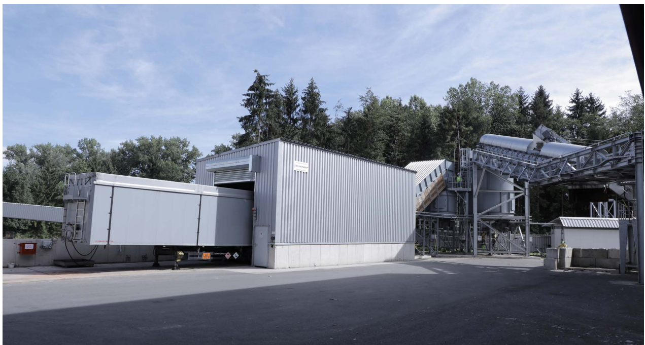
Picture 2: The BG OptiBulk unloading station is equipped with a special housing, which protects the environment from dust escape and the material from environmental stress.
