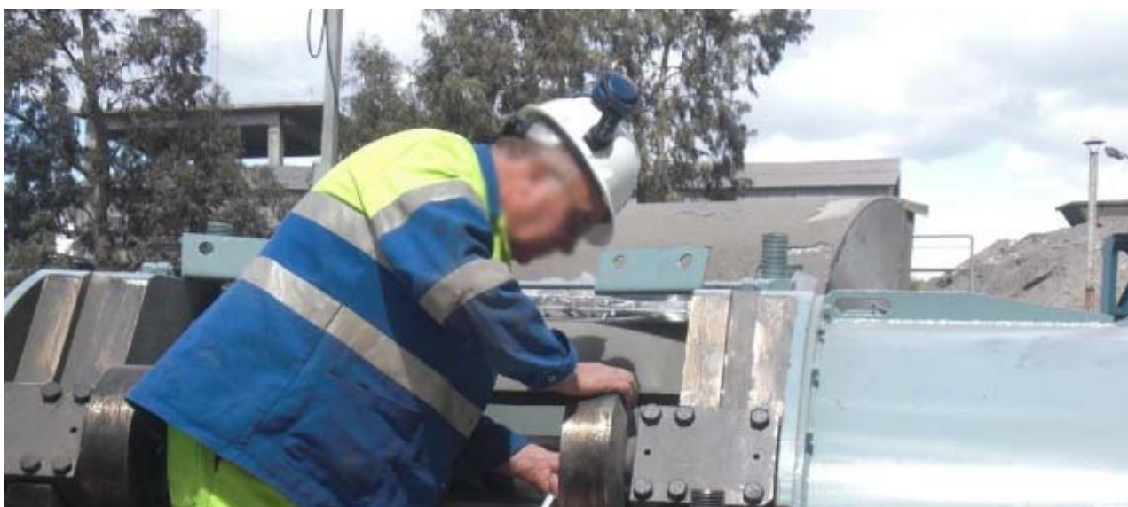
Fig 9 –Kiln upgrade with Bogiflex® KGD26
