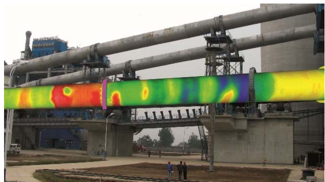
Fig 2 – Thermal readings of running kiln
