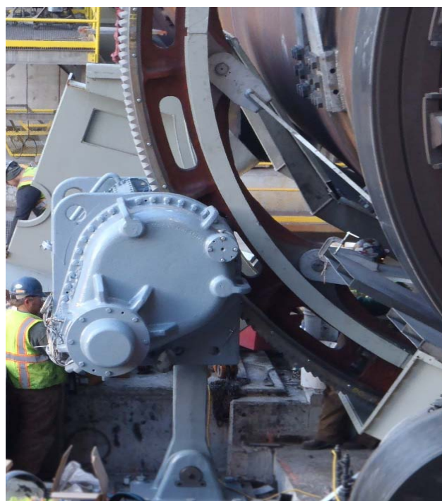
Fig 10 – example of Bogiflex® KGD20 during installation
