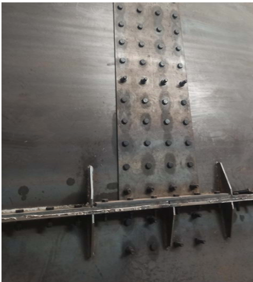
Silo wall plates connection points
