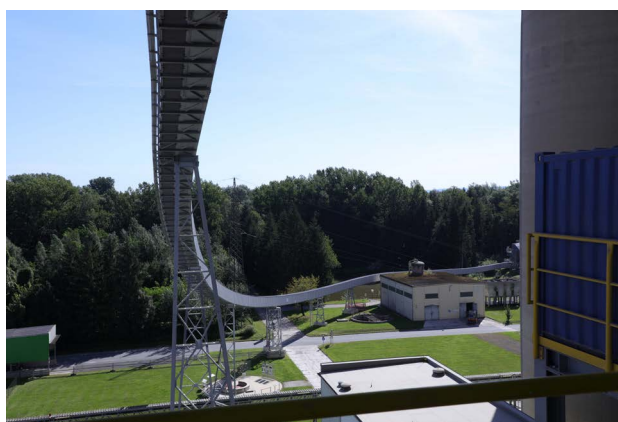
Picture 5: Inside of a U-shape conveyor
