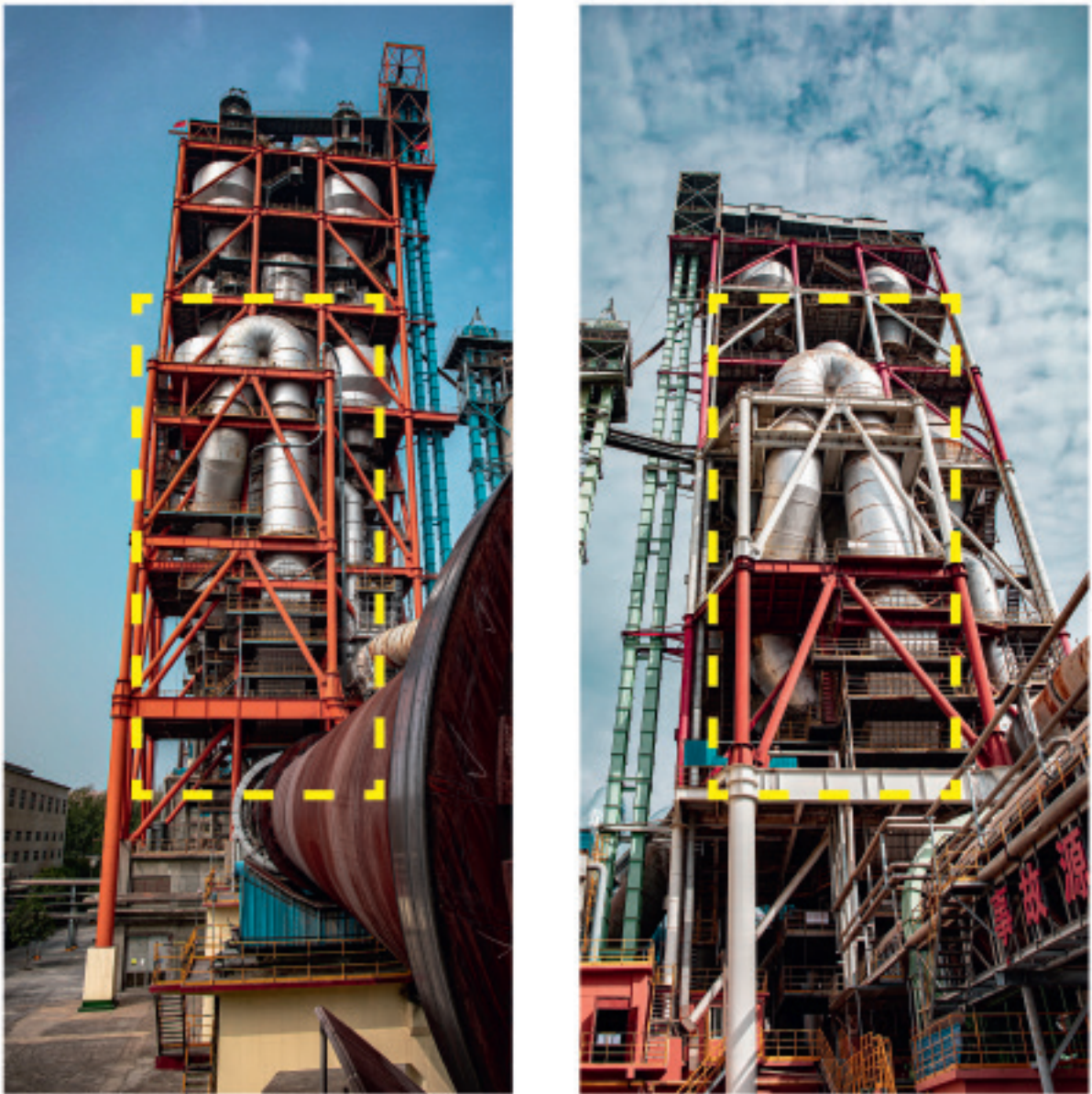
Figure 8: Pyroredox installations in China.
