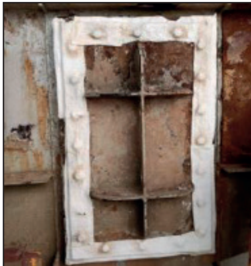
Fig 05: Conventional False Air arresting methods (By Ceramic Paper + Sodium Silicate)
