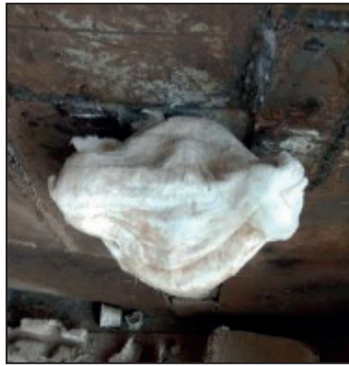
Fig 05: Conventional False Air arresting methods (By Ceramic Paper + Sodium Silicate)
