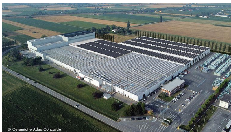
Aerial view of the extended area of the Finale Emilia site
