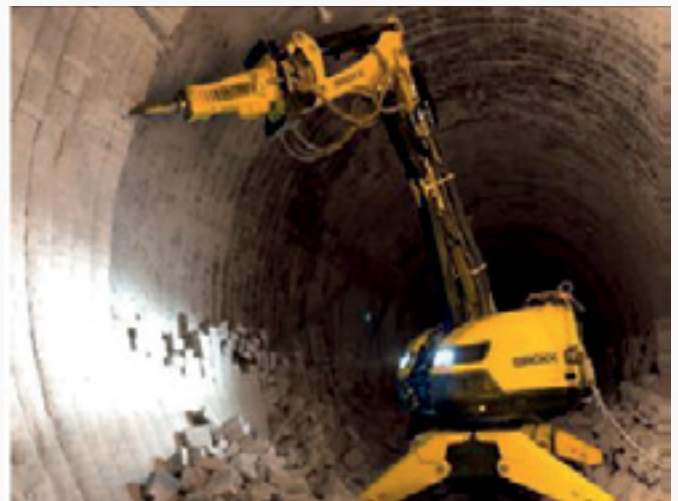
A demolition robot working in a kiln is remote controlled.
