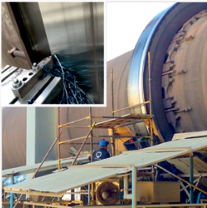
Figure 8: Insitu tyre machining at 3,5 rpm.
