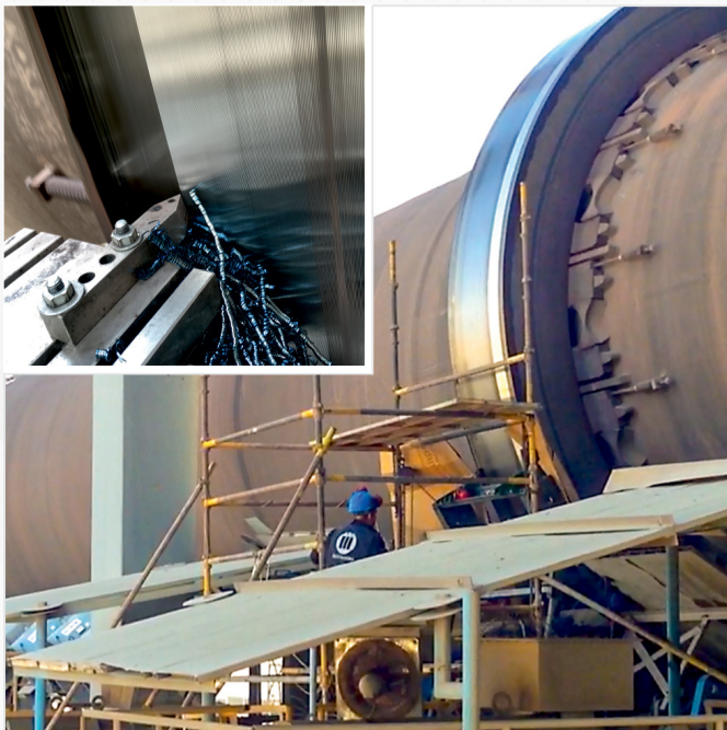
Figure 8: Insitu tyre machining at 3,5 rpm.
