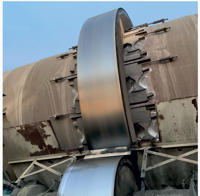
Figure 7: Insitu machined and grinded tyre and roller.
