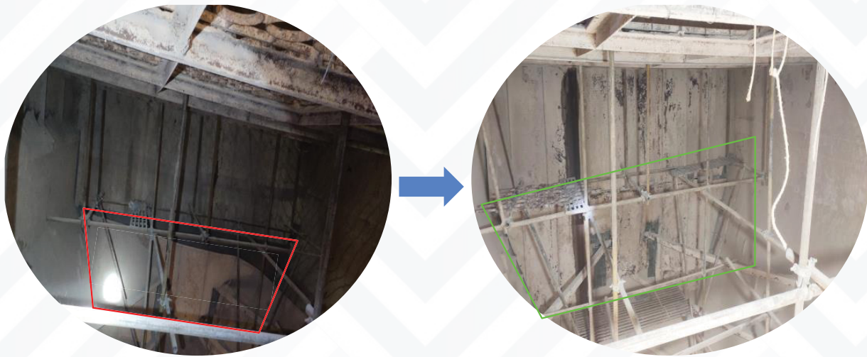
Baffle plate repair
