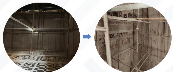
Bottom grid removal
