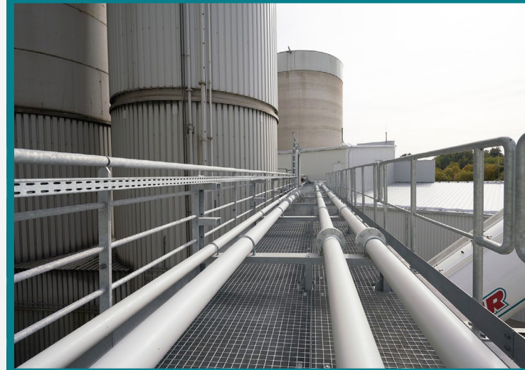
Feeding of various alternative fuels to rotary kiln
